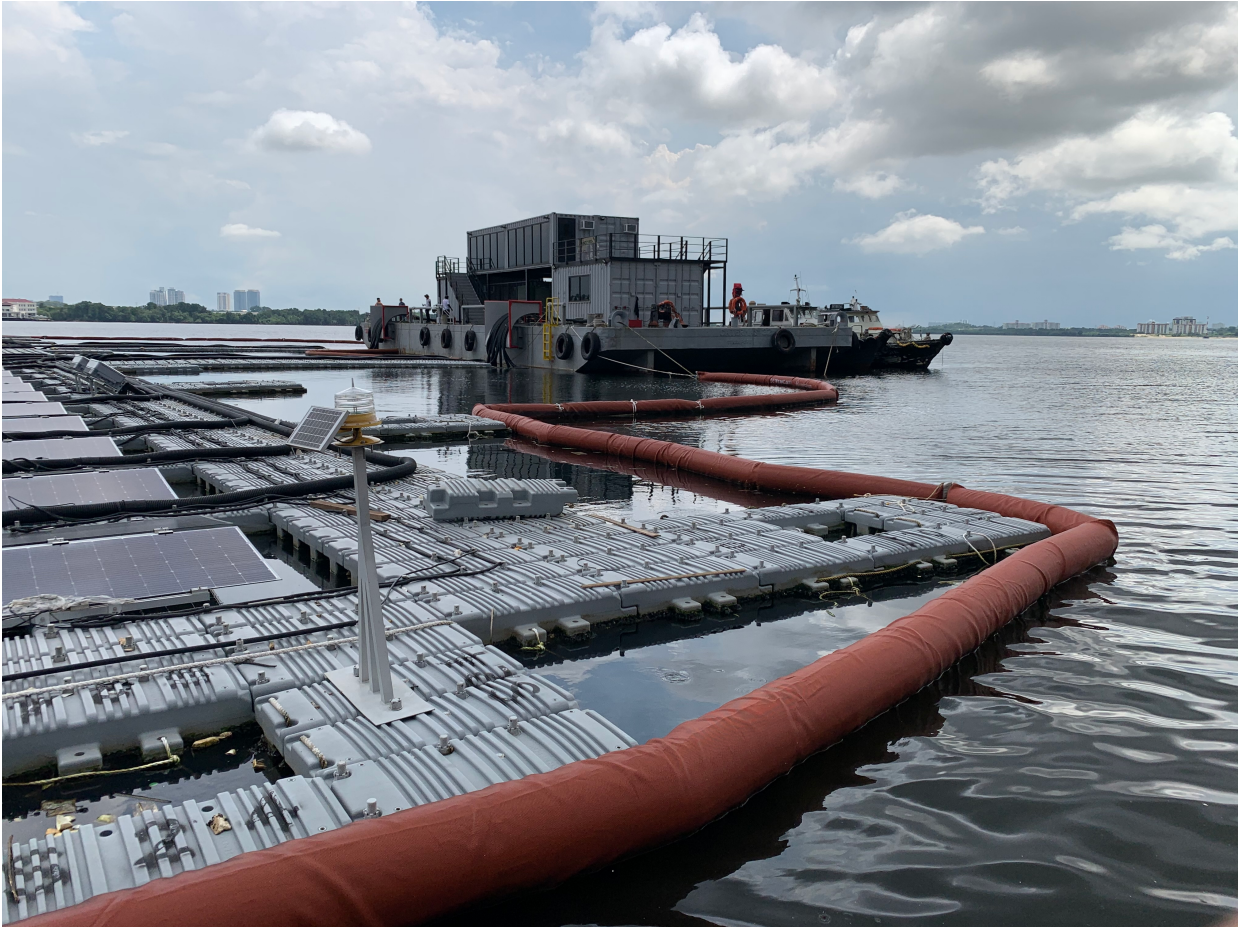
Figure 3: Debris Barrier installed around the solar farm
