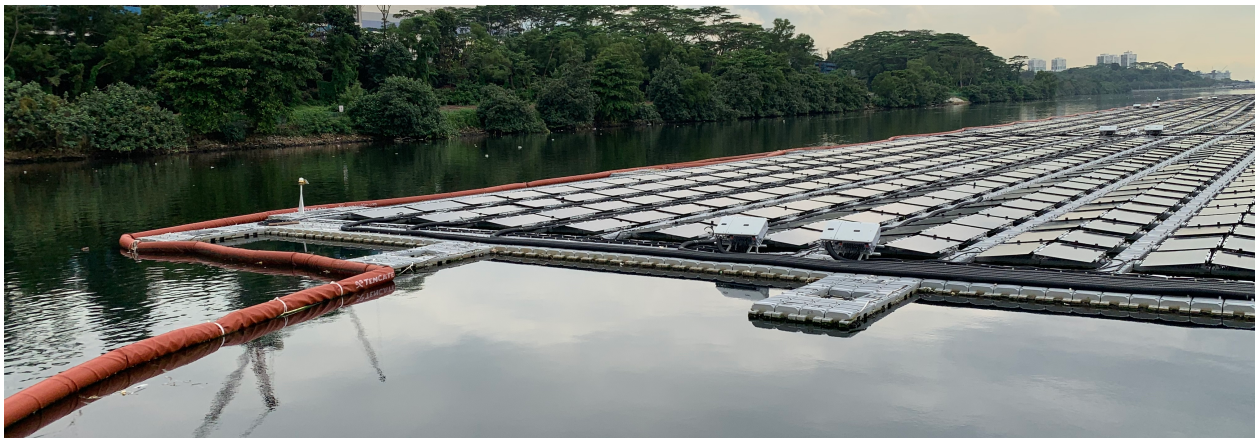
Figure 5: Debris Barrier installed along the perimeter the solar farm
