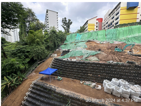
Figure 2: Layers of Geobags installed in the multi terrace GeoBarrier system.
