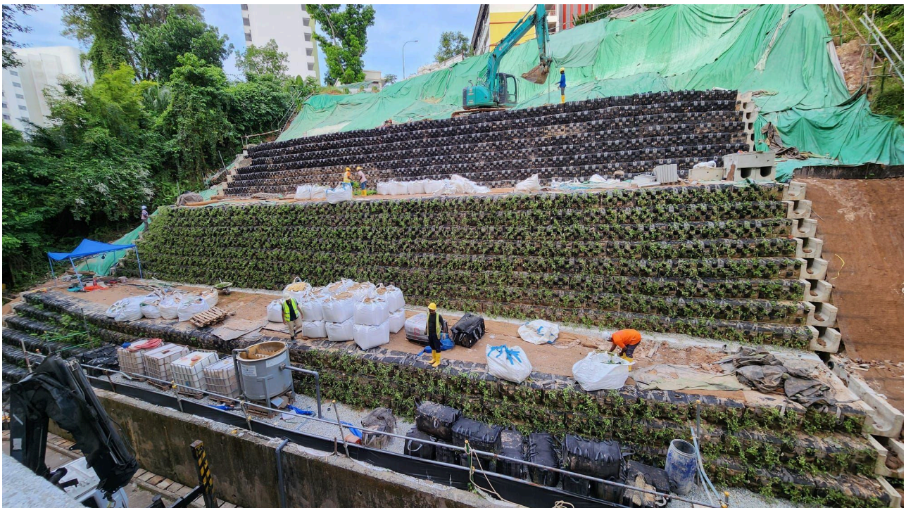
Figure 5: Utilising the working platforms to store materials and access for machinery.
