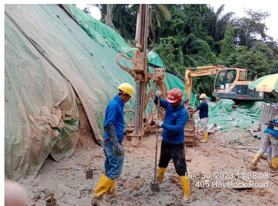
Figure 3: Installing the ground lock system
