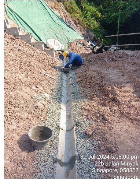
Figure 4: Constructing the surface run off drains at the toe of the terrace.
