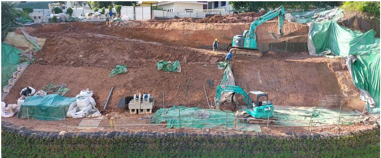
Figure 6: Excavators delivering materials from the crest of the slope to the respective working platforms
