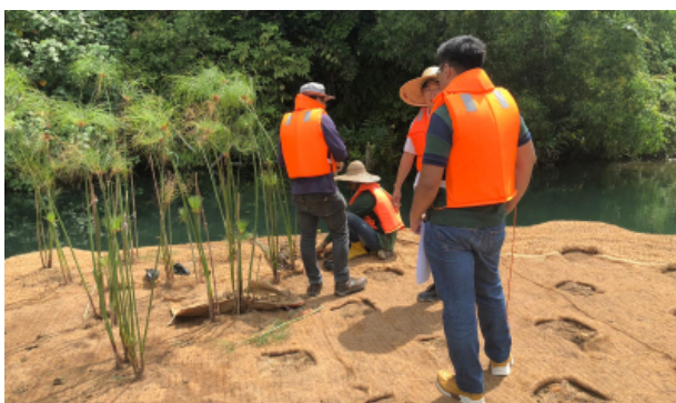
Figure 22: Planting the plants on the floating platforms
