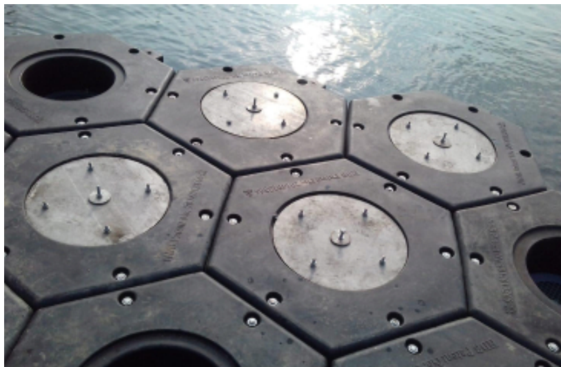
Figure 8: The mooring bracket installed on the floating modules
