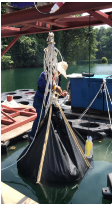
Figure 17: Using the winch to lower the sinker.
