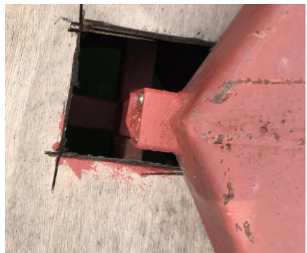
Figure 13: The anchor system of the floating crane to the floating platforms is covered with plywood, creating a secure and stable structure
