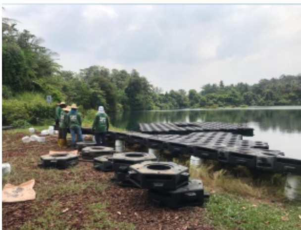
Figure 3: Assembling the floating modules
