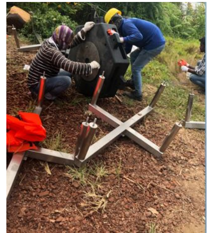
Figure 7: Installing the Mooring system.
