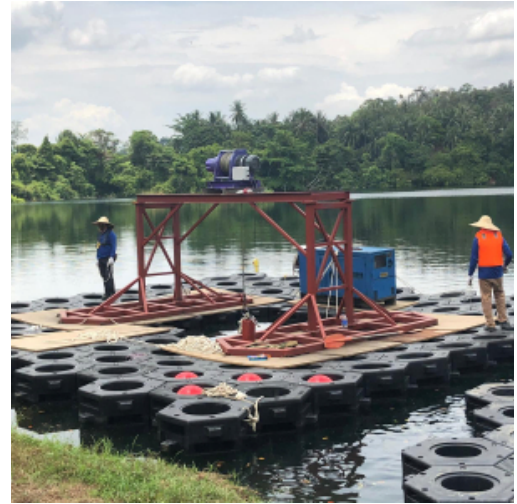
Figure 11: Installing the Floating crane
