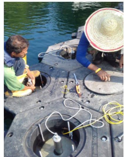
Figure 9: Installing the mooring bracket
