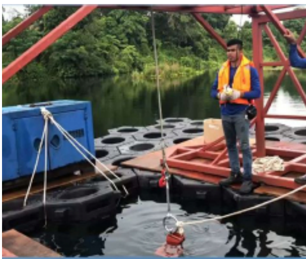
Figure 12: Running trial test on the winch system.
