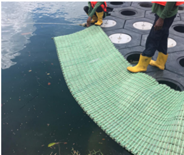
Figure 19: Installing the floating mat.
