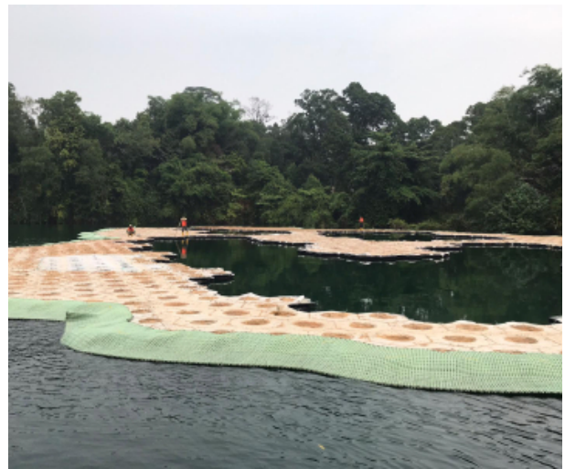
Figure 21: Earthfilling carried out on the floating platform
