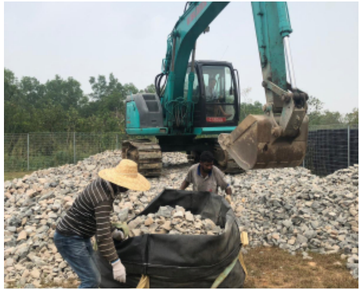
Figure 15: Using Hydraulic Excavator to fill the Geosynthetic bags with granite.
