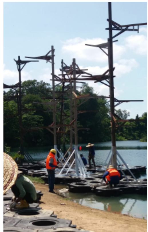
Figure 27: Installing of the Nesting Structure onto the floating platform
