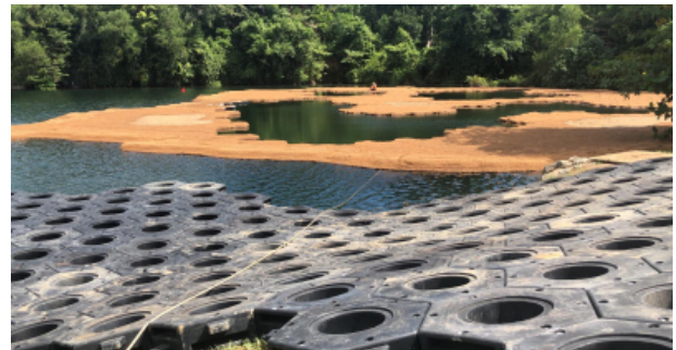
Figure 18: Covering the floating modules with geotextile.
