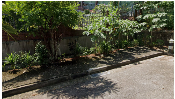
Figure 1: Cheng Soon Garden's retaining wall before the collapse
