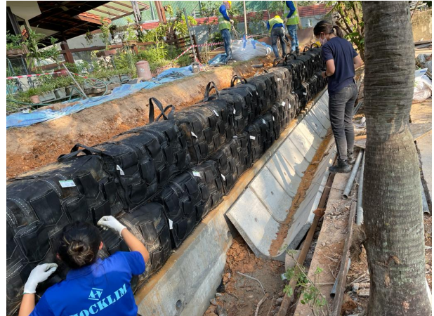
Figure 7: Engineers ensuring the bags are compacted properly
