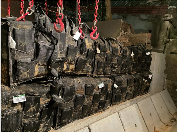
Figure 6: Building of the GeoBarrier System
